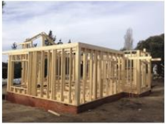
Fig. 1. Timber frame structure Source 1: 100x100 Madera
