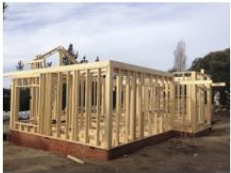
Fig. 1. Timber frame structure Source 1. 100x100 Madeira
