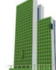
HoHo Vienna Vienna, Austria 24 Stories Under Construction 2018
