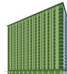
Brock Commons Tallwood House Vancouver, Canada 18 Stories 2017
